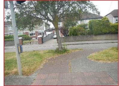
On the western side of the crossing the stem of the tactile paving should terminate at the location where the footpath changes direction. Buff coloured tactile paving, 1.2m deep, should be provided at the existing dropped kerb and a new dropped kerb provided on the other side of the service road with a similar tactile paving arrangement, ensuring the dropped kerbs and tactile paving are aligned.
