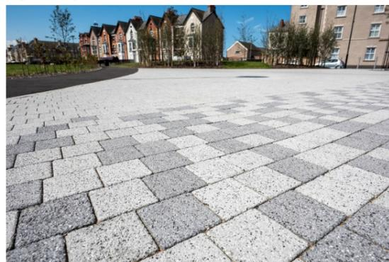
**Fig. D Concrete paving with textured finish**
